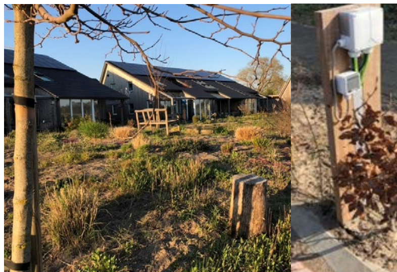
Fig 2. (a) Vriendenerf community houses, (b) moving towards e-mobility: the first EV charging infrastructure. These chargers are to be upgraded at a later stage to controllable EV chargers (11kW) 1 [Saxion, 2022]
